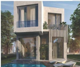
VILLA (C) // BACK FACADE
