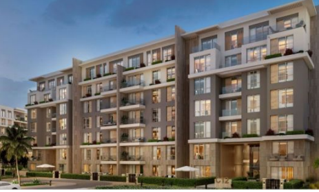
Building Type 3 - Front view
