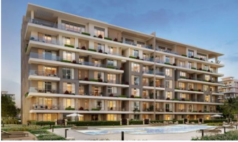
Building Type 3 - Back View
